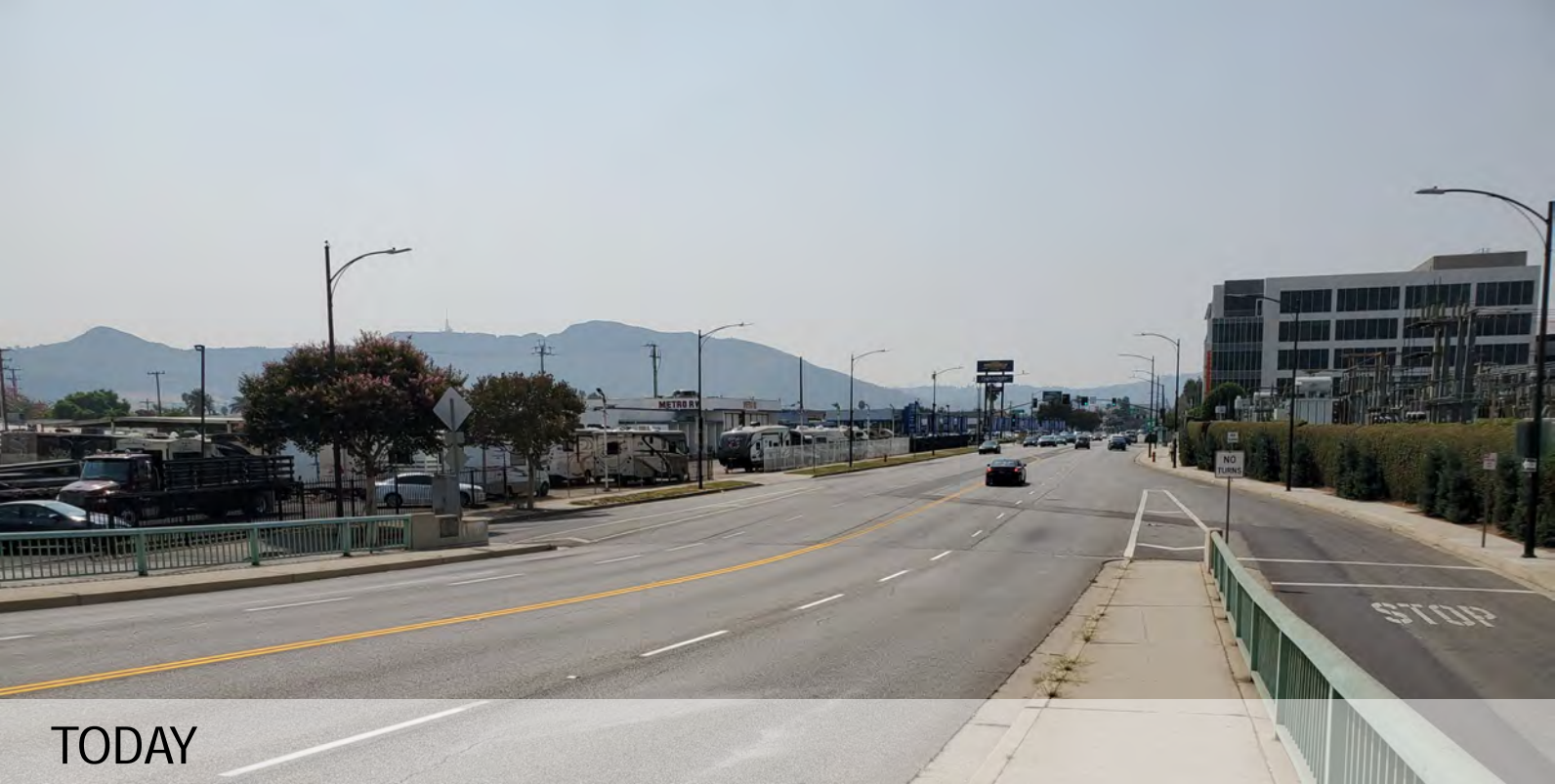
OLIVE AVENUE DISTRICT
