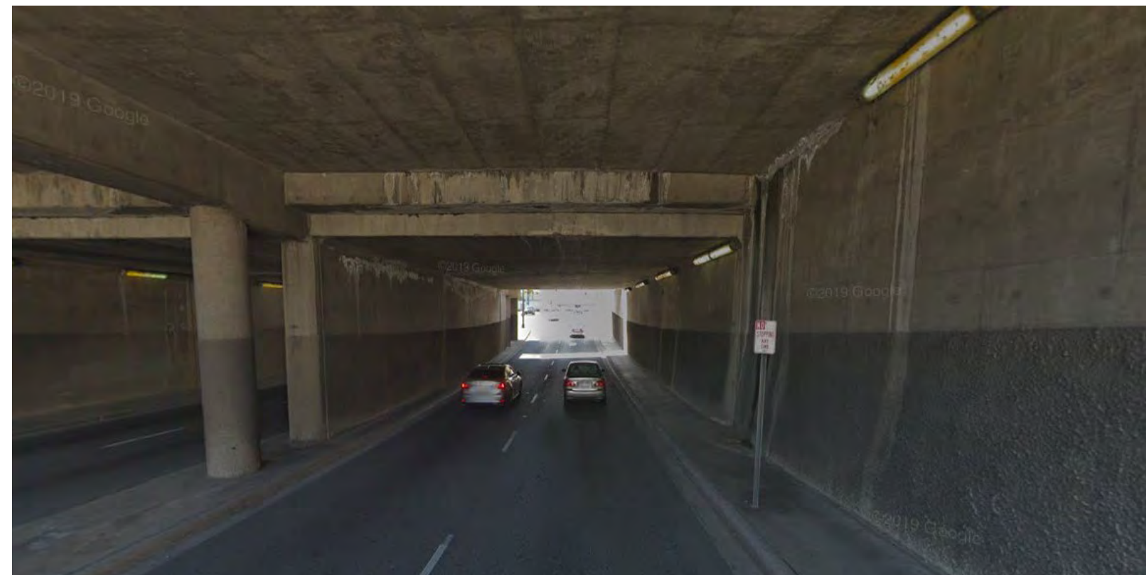
ALAMEDA AVENUE I-5 UNDERPASS
