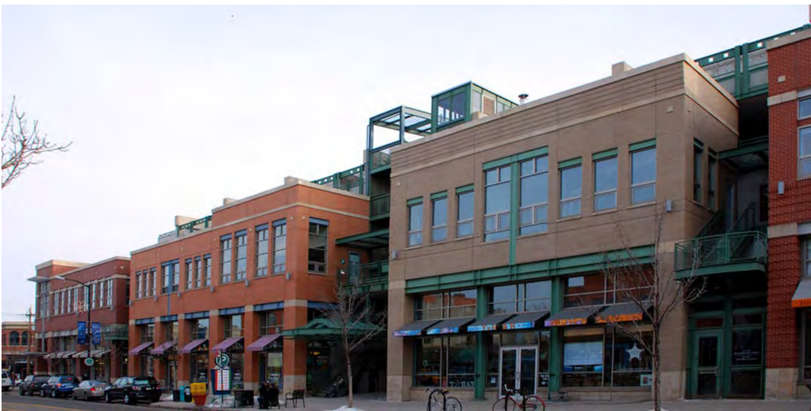
LINED PARKING STRUCTURE
