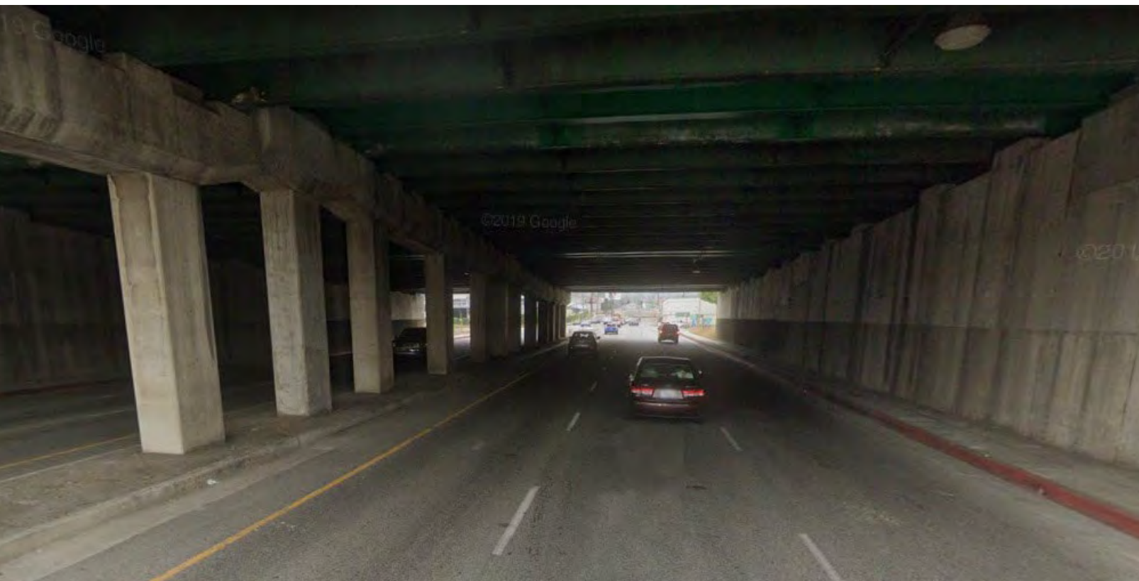
ALAMEDA AVENUE RAILROAD UNDERPASS
